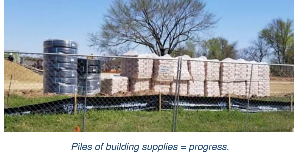
Piles of building supplies = progress.
